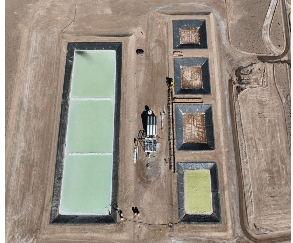
Aerial view of original HMW Pilot Plant
