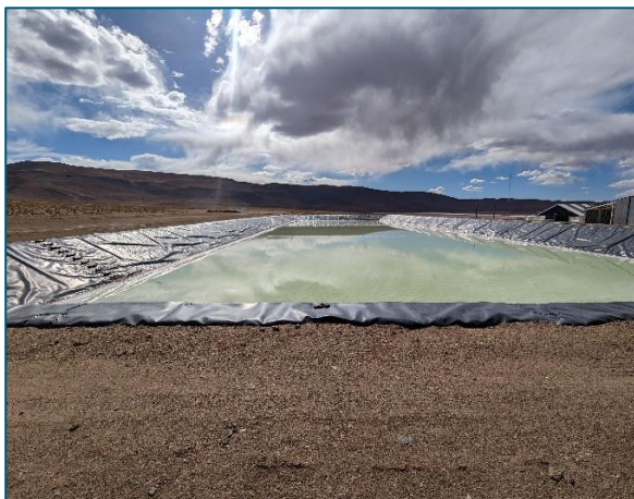
Figure 26: Test pond 1 (3000m 2 ) – Brine pumped to next pond when it reaches ~0.4% Li
